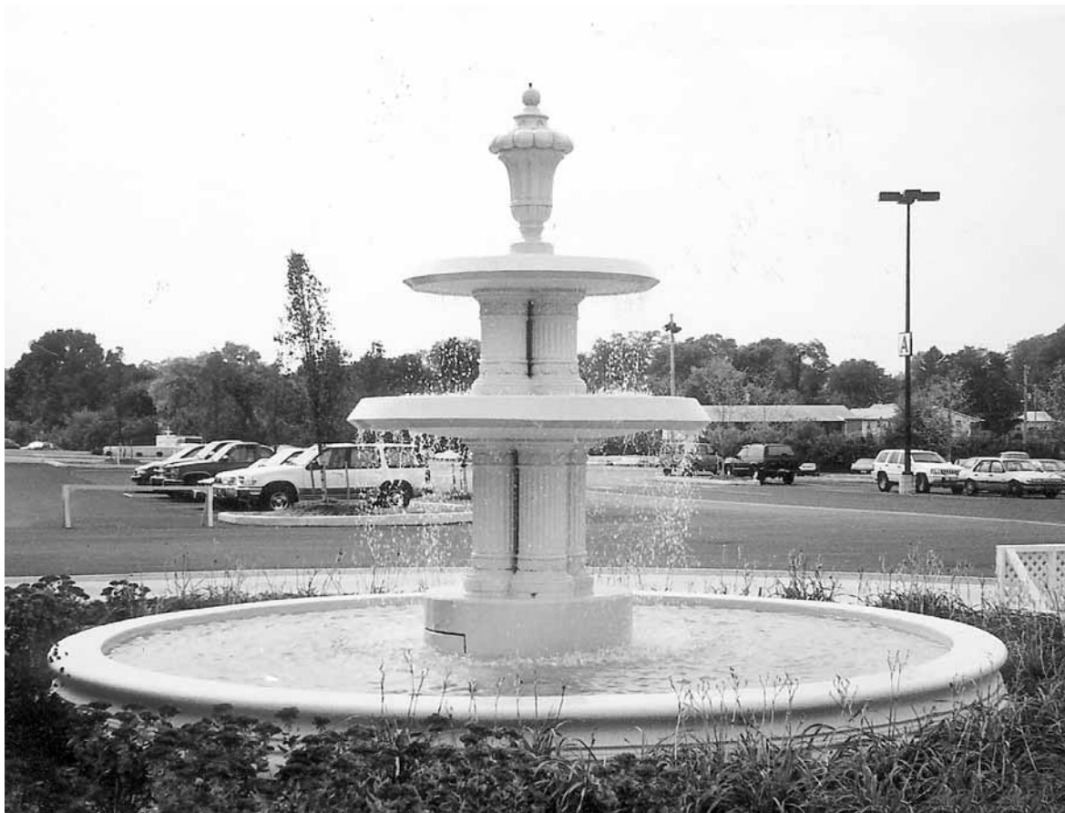
FOUNTAIN AT THE CHARLESTOWN RACE TRACK in Charlestown, West Virginia Architectural Concepts designed for Warfel Construction.
